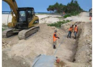
Preparing to install gabions at Dry Creek, from left to right, Rose David, "Pin" Chandra and Wesley Timas check the dimensions of the excavation. In the background Joshua Matai makes up the wire gabion baskets.
