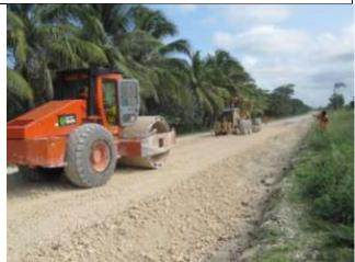
Downer roller and grader compacting and shaping pavement at Banana Bay. On the right Abel Reynolds uses a level to check the pavement as it is laid.
